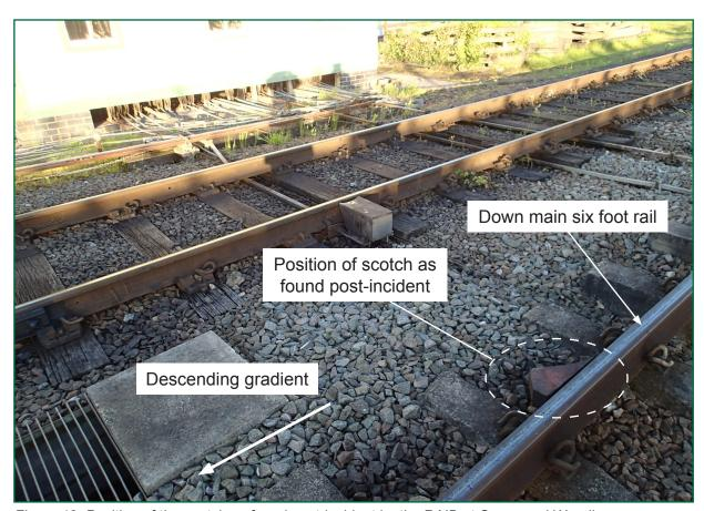
Figure 12: Position of the scotch as found post-incident by the RAIB at Quorn and Woodhouse
