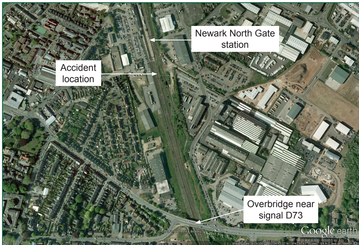
Figure 2: Google earth image of the accident site
