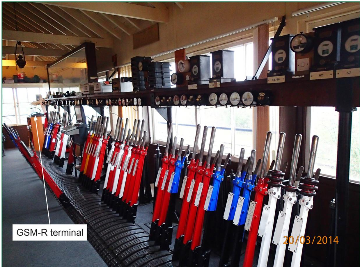
Figure 4: interior of Greenford signal box, showing lever frame.
