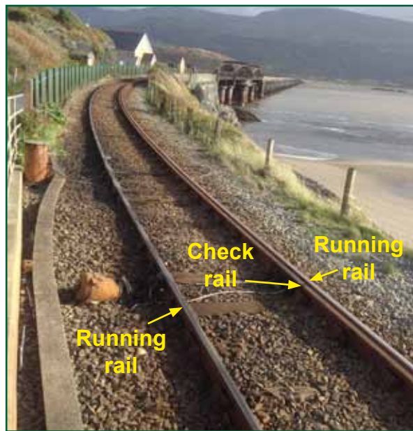
Figure 13: Typical check rail
