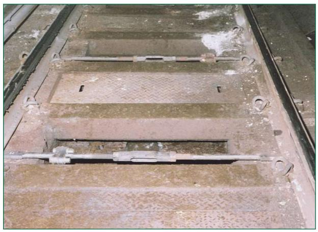
Figure 3: Tie-bars fitted to the track close to where the derailment occurred (courtesy of British Transport Police)
