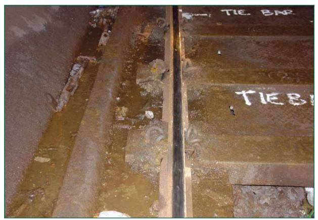
*Figure 5: Showing the degree of contamination around housings and locations marked for further fitment of tie-bars*
