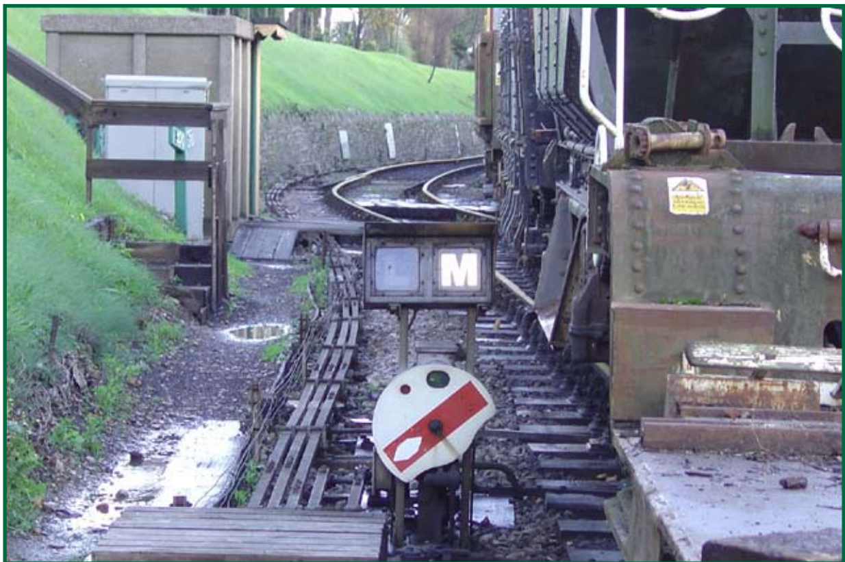
Figure 5: Signal 25 as seen looking towards Swanage station. The 'M' indication is displayed
