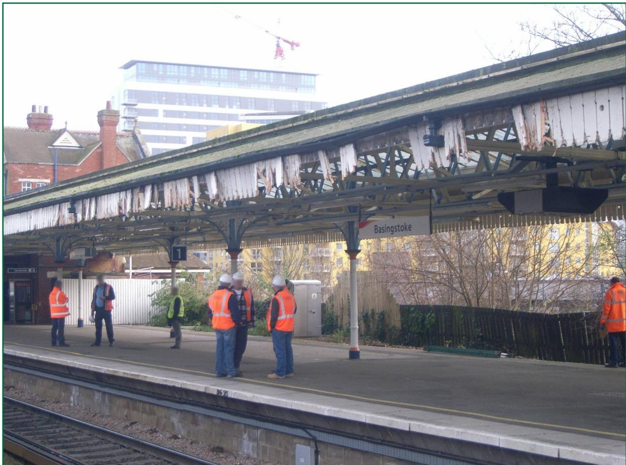
Figure 2: Canopy of platform one, Basingstoke, showing damage
