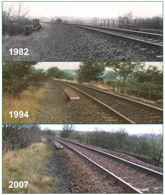
*Figure 17: The level of ballast on Bridge 88 when photographed for assessments in 1982, 1994 and 2007 (photographs courtesy of Network Rail)*
