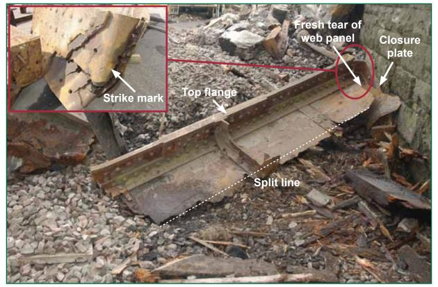
Figure 12: Upper part of the south end of the centre main girder showing the horizontal split line, the folded closure plate and fractured flanges (main photograph courtesy of British Transport Police)
