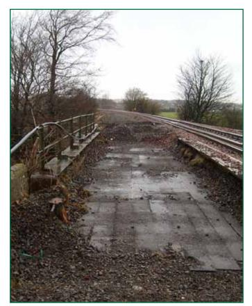
Figure F3: Site photograph of the west deck after the ballast was removed on 16-17 January 2009 (photograph courtesy of Network Rail)
