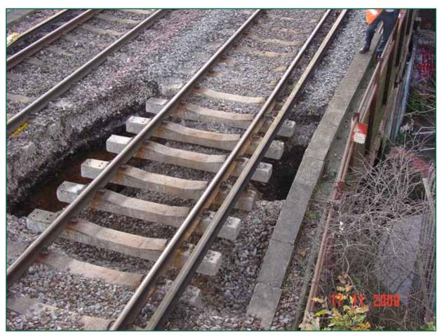
Figure 7: Overview of track showing loss of support to up line
