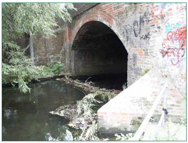
Figure 4: Branch across upstream face of bridge 48 on 20 August 2009 (photograph: N Banks)
