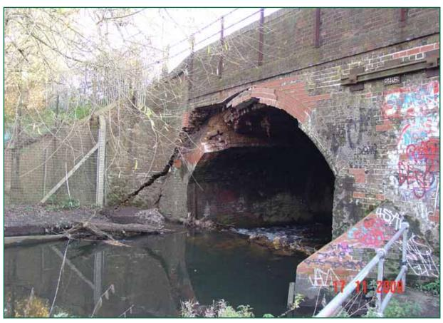
Figure 6: upstream face of bridge 48 following the incident showing failed arch
