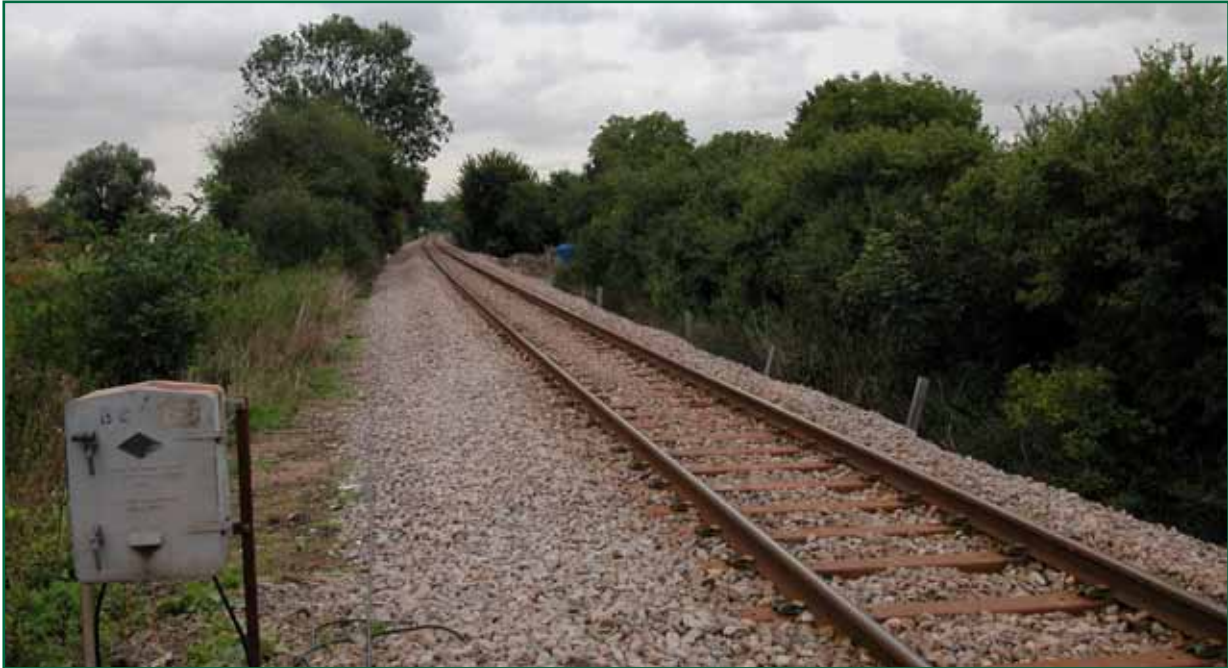
Figure 5: View from Sewage Works Lane UWC looking towards Shalfords UWC and Sudbury.
