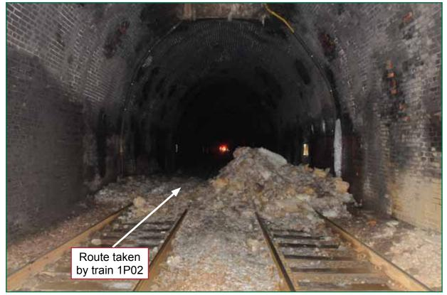
*Figure 8: General view of the pile of ice found below ventilation shaft 10 after the accident (courtesy of British Transport Police)*
