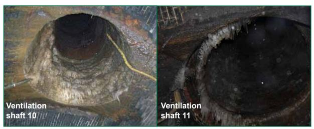
Figure 11: Views looking up at ventilation shafts 10 and 11 showing ice still present in the bottom of the shafts (ventilation shaft 11 photograph courtesy of British Transport Police)
