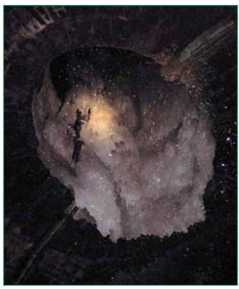
Figure 15: The ice formation seen hanging from the bottom of a ventilation shaft in Blea Moor tunnel in December 2010 (courtesy of Network Rail)
