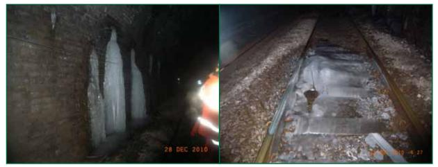
Figure 12: Ice formations found on the track and tunnel wall
