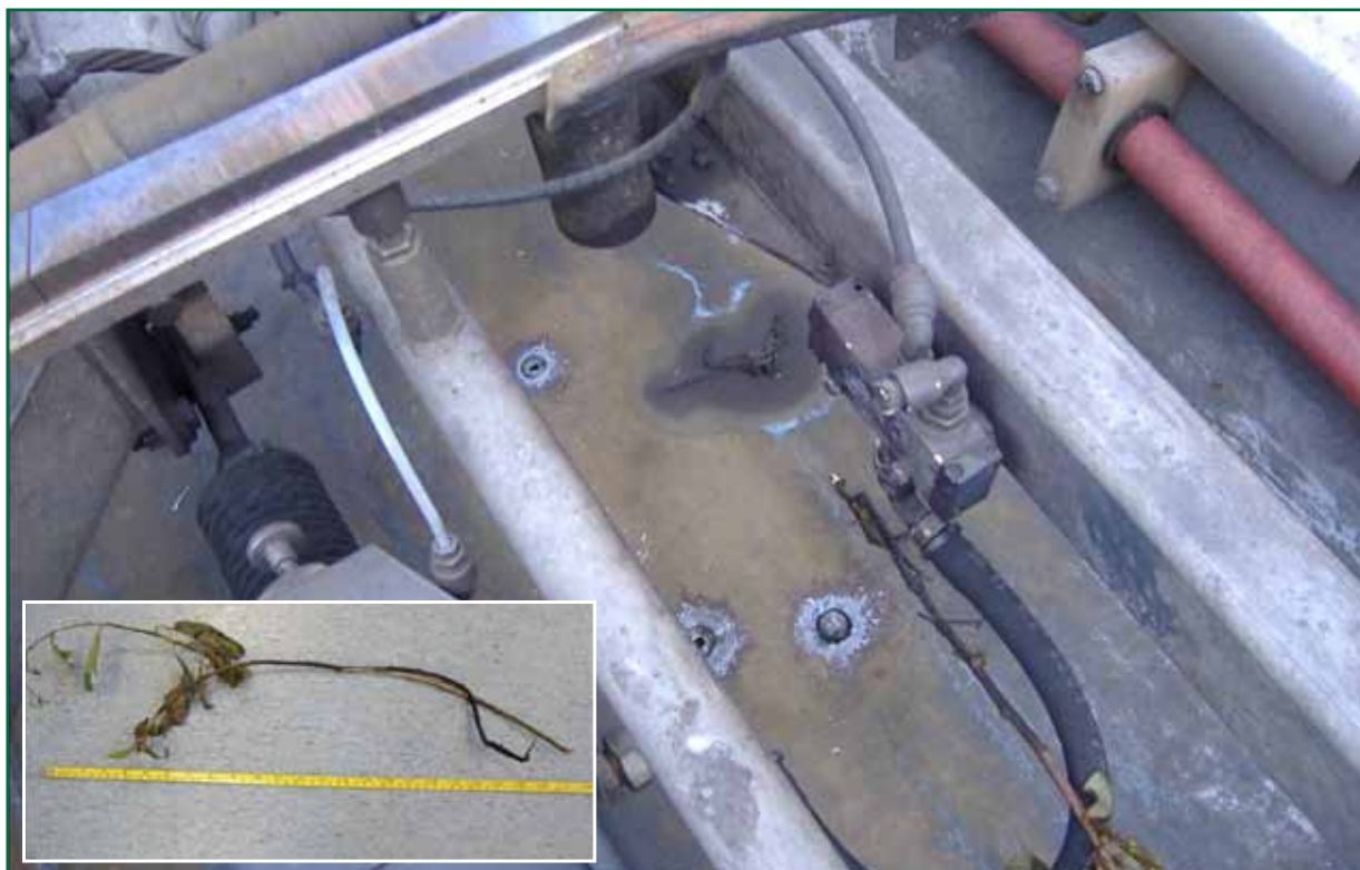
Figure 5: Damaged pantograph with foliage
