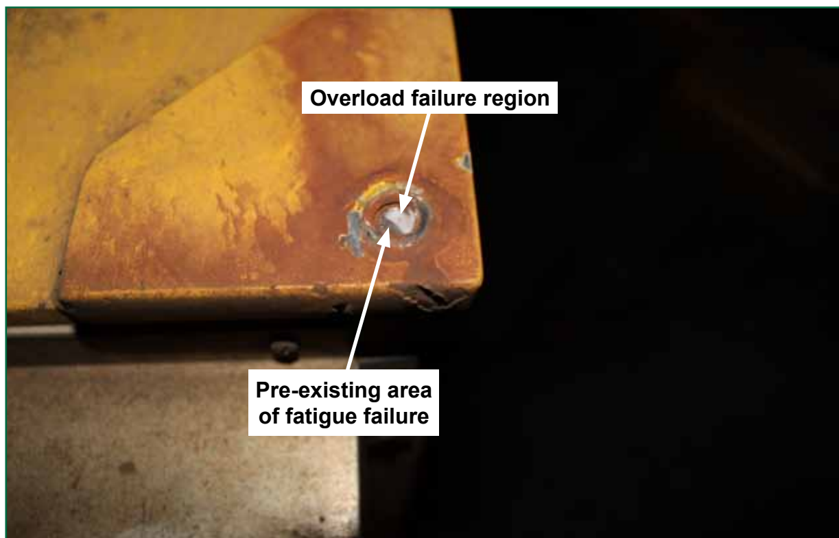
Figure 12: Lower section of bolt F1 (inserted into cab roof) showing evidence of pre-existing fatigue and final overload fracture
