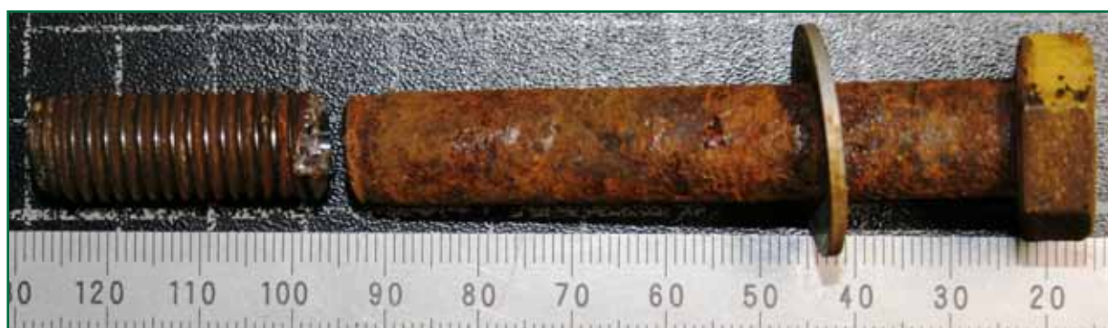
Figure 17: Corrosion on bolt R3
