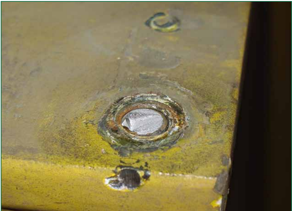
Figure 11: Lower section of bolt R4 (inserted into cab roof) showing clean-break indicating overload failure of the bolt
