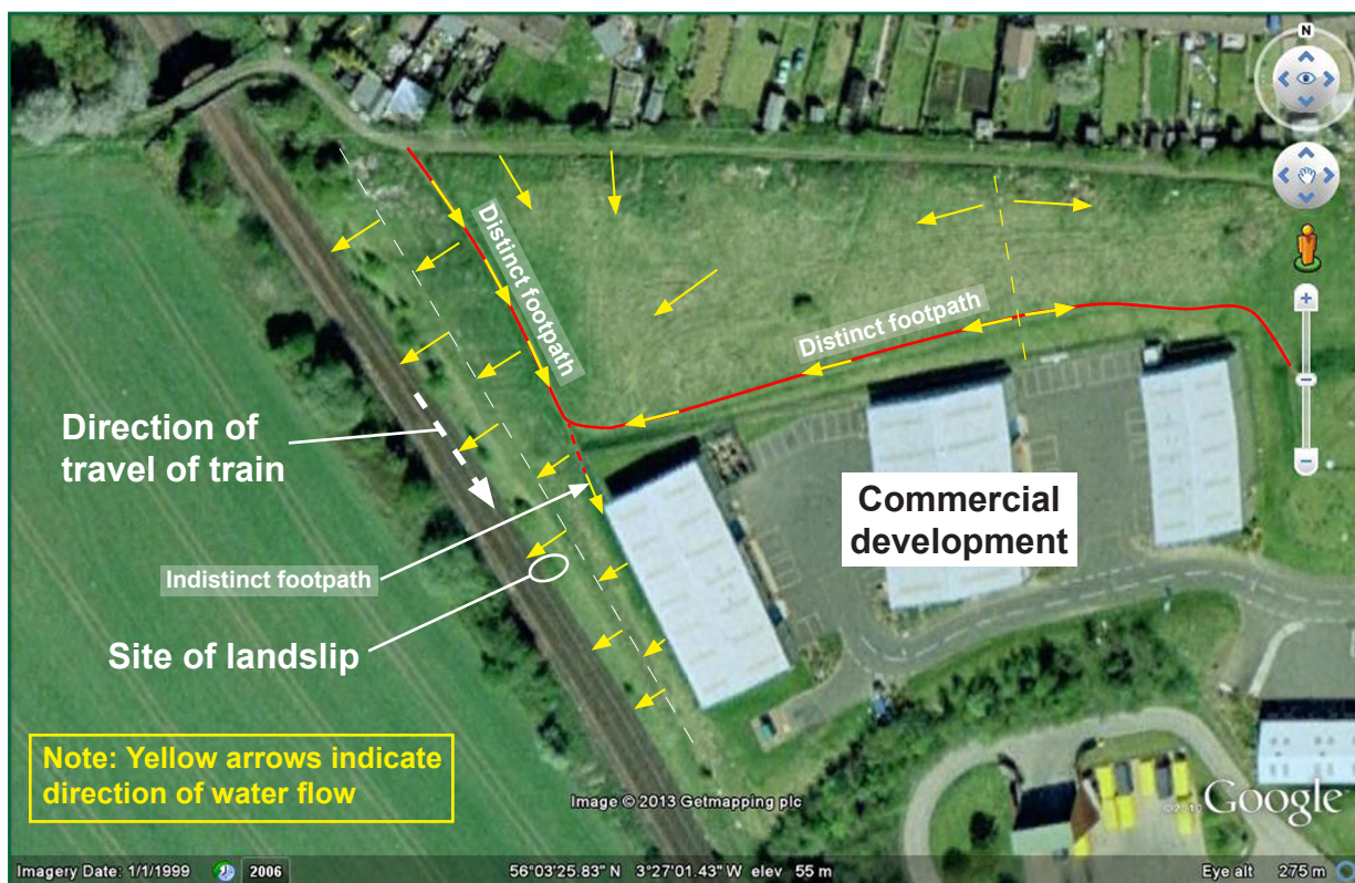
Figure 16: Rosyth: landslide and surrounding land features (pre-incident photograph)
