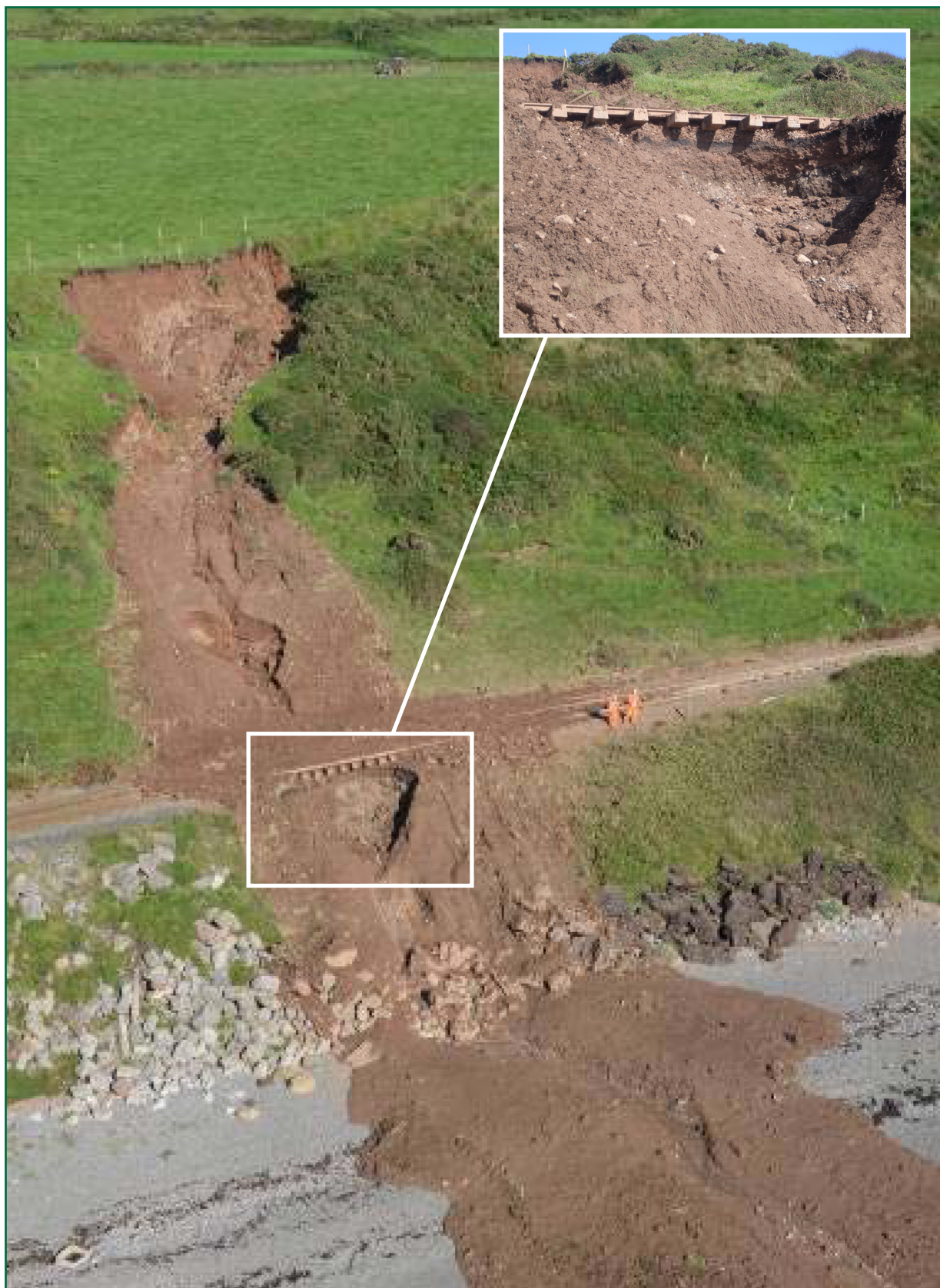
Figure 19: St Bees: landslide at 68 miles 59 chains (main image courtesy of Network Rail)
