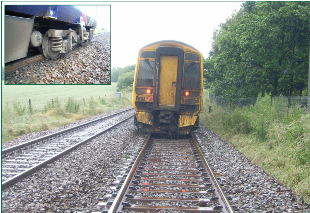
Figure 14: Rosyth: derailed train
