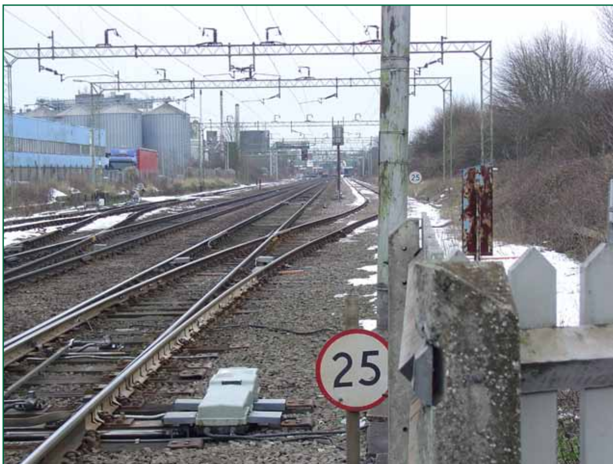
Figure 5: View from north-west (down) side of Motts Lane crossing, looking towards Witham station
