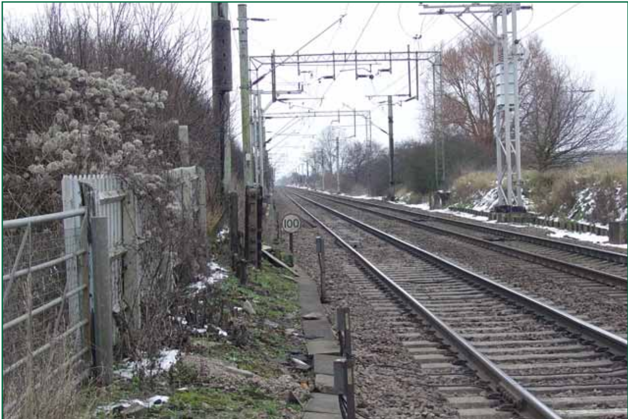
Figure 6: View from north-west (down) side of Motts Lane crossing, looking towards Kelvedon station
