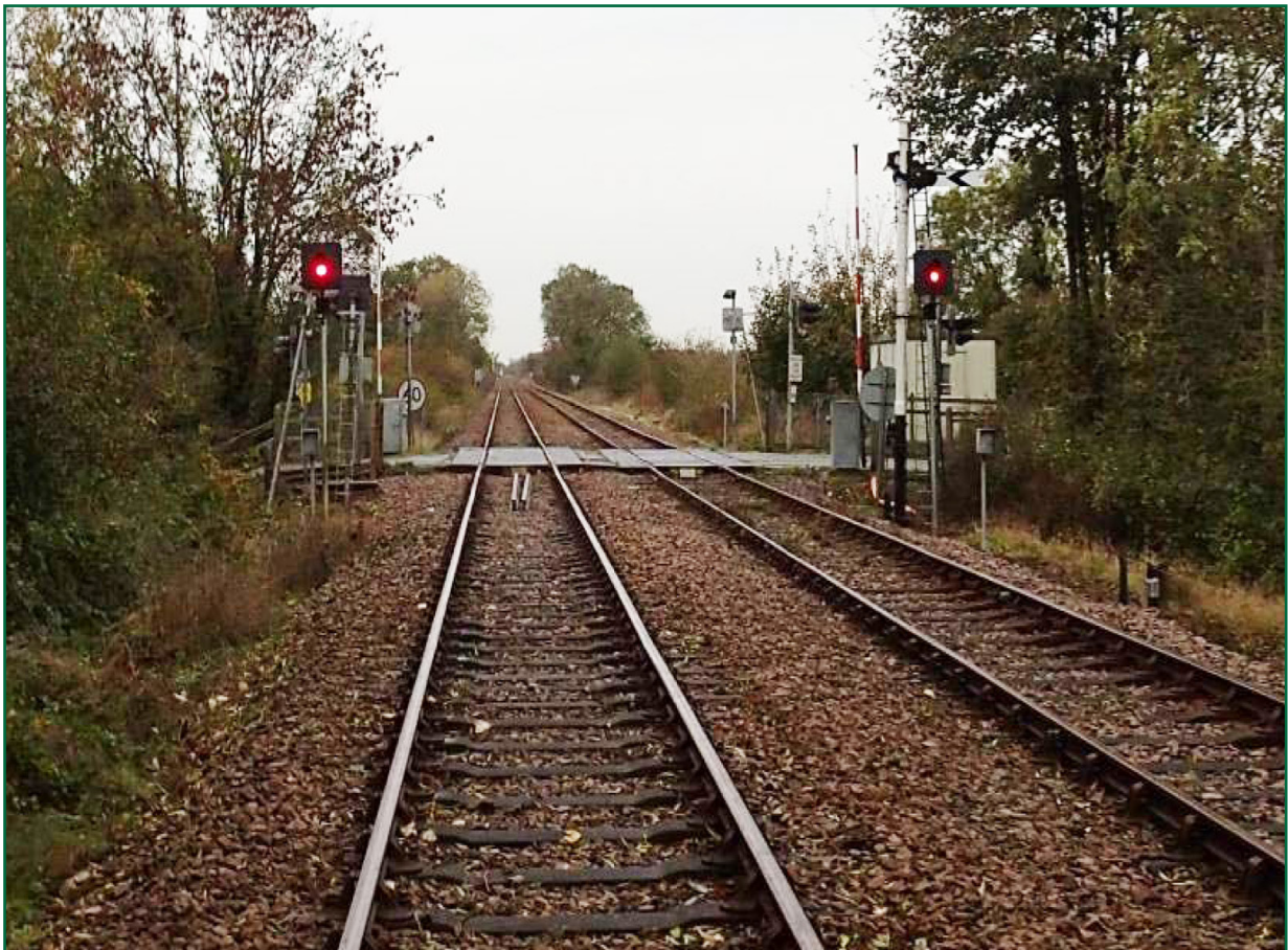
Figure 4: Butterswood ABCL level crossing - rail approach
