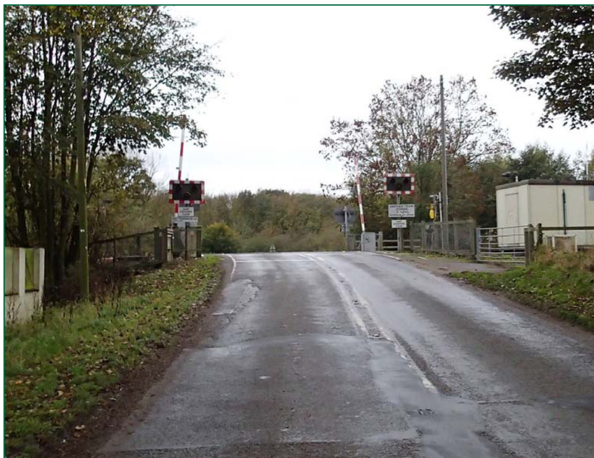
Figure 3: Butterswood ABCL level crossing - road approach
