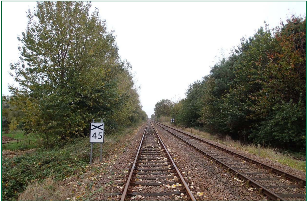
Figure 6: The special speed restriction board, around 303 metres from the level crossing
