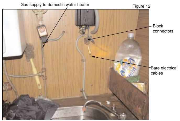
Example of block connector use and exposed wiring
