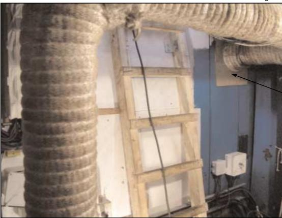
Area of bulkhead penetration. (Now shown with a post repair closure plate.)
