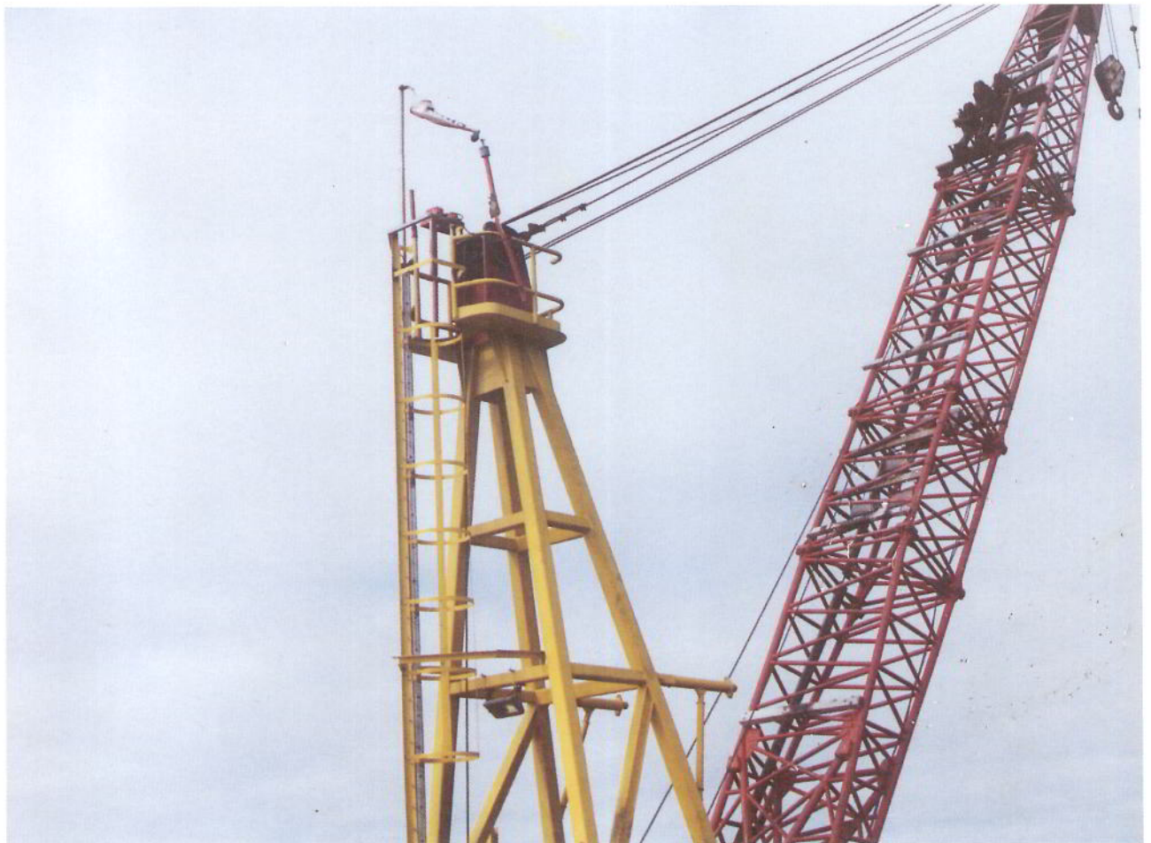
Damage to Brent Spar helideck and crane "A" frame.
