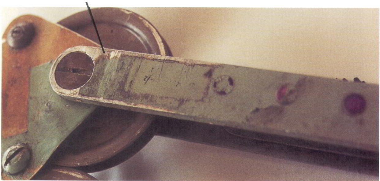
PHOTO 4.1 - RIGHT AFT DIFFERENTIAL PULLEY LEVER
