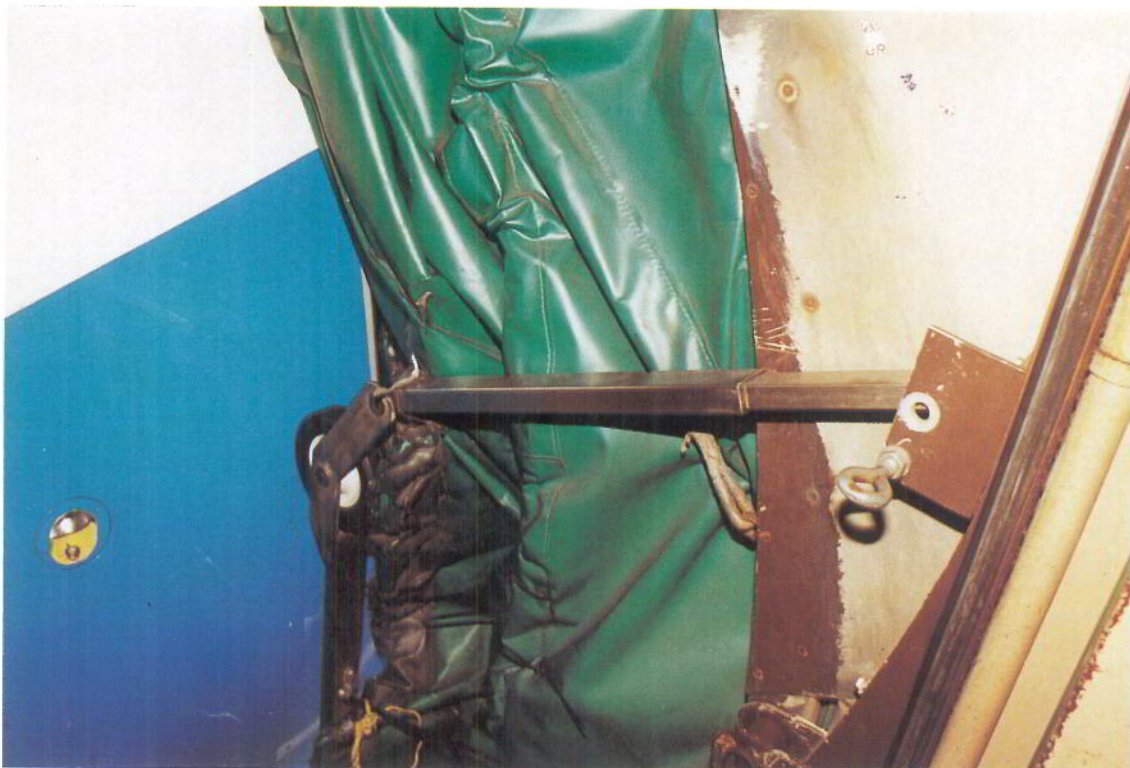
Rearwards railing and idler wheel contacting skin. Note telescopic rail and proximity of rectangular section outer tube end to adjacent structure.
