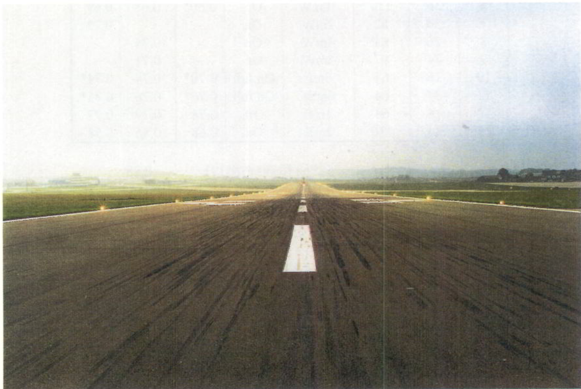
Figure 7 Rubber deposits at runway 34 threshold
