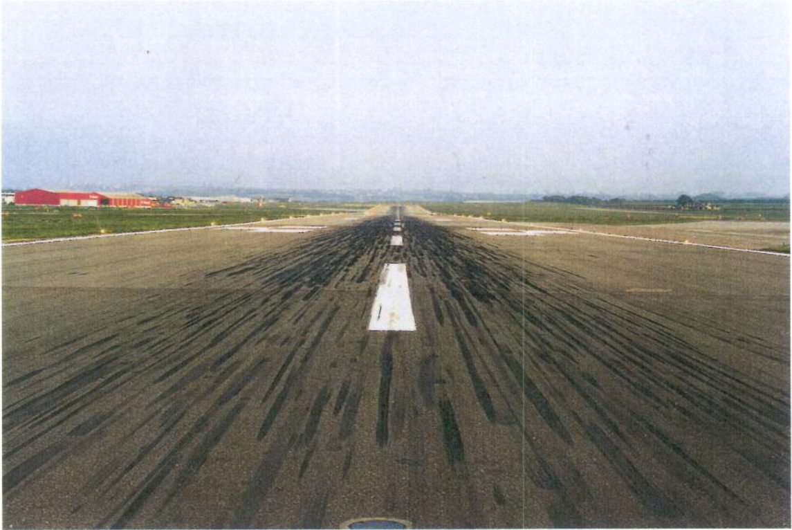
Figure 6 Rubber deposits at runway 16 threshold
