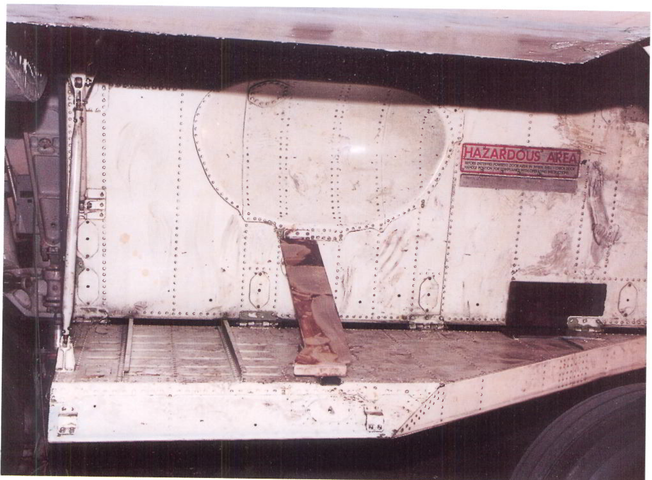
PHOTO 2 DOOR SLIDE RAMP FITTED TO RIGHT HAND BODY GEAR DOOR
