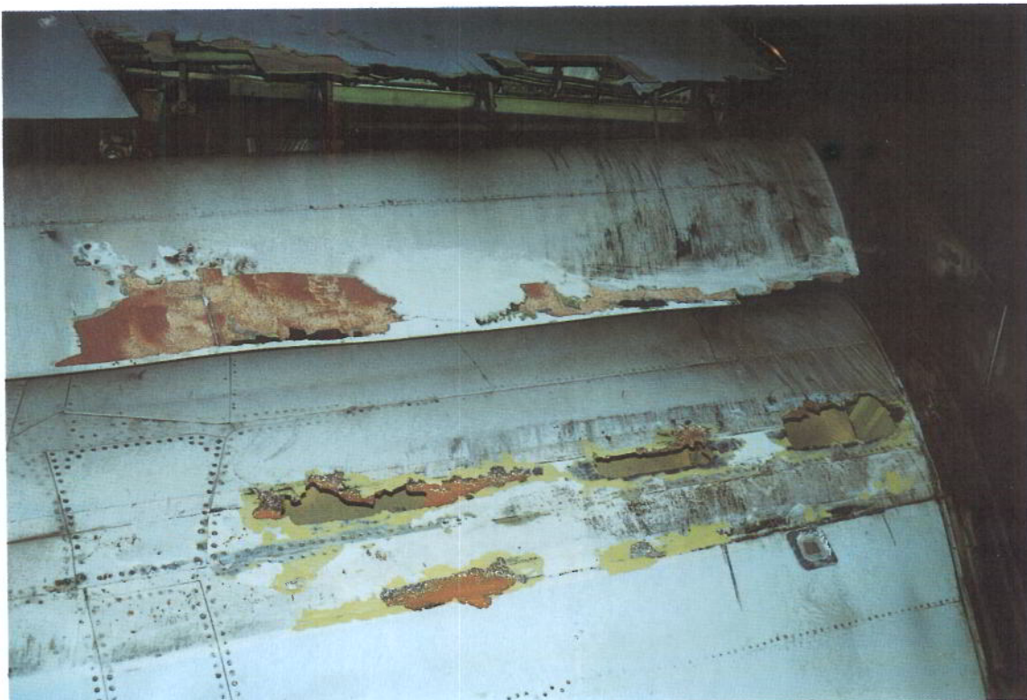
G-BDXH - Damage to mid-and fore-flap due to break-up of trailing edge panel
