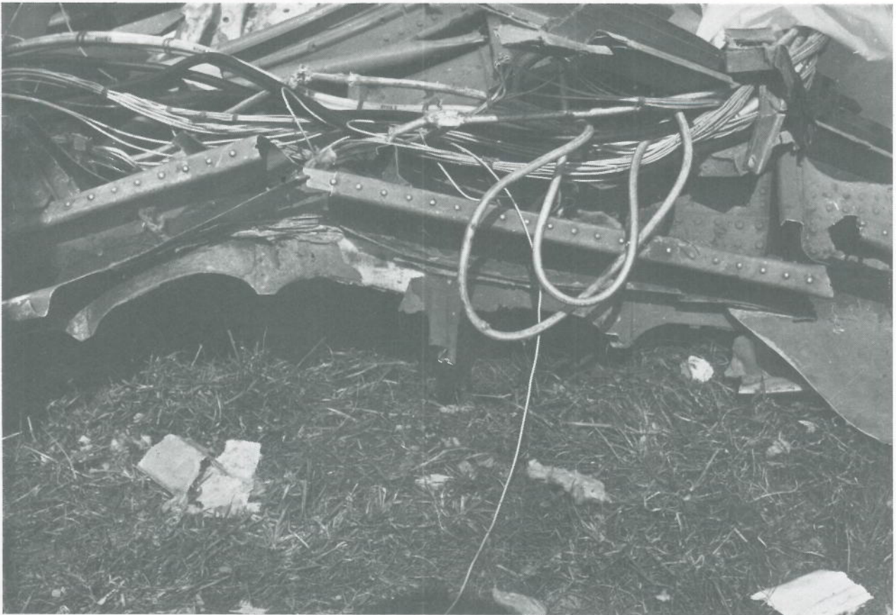
Figure n° 7: Lower portion of fuselage station 1223, showing severe corrosion attack and delamination in the rear pressure bulkhead.
