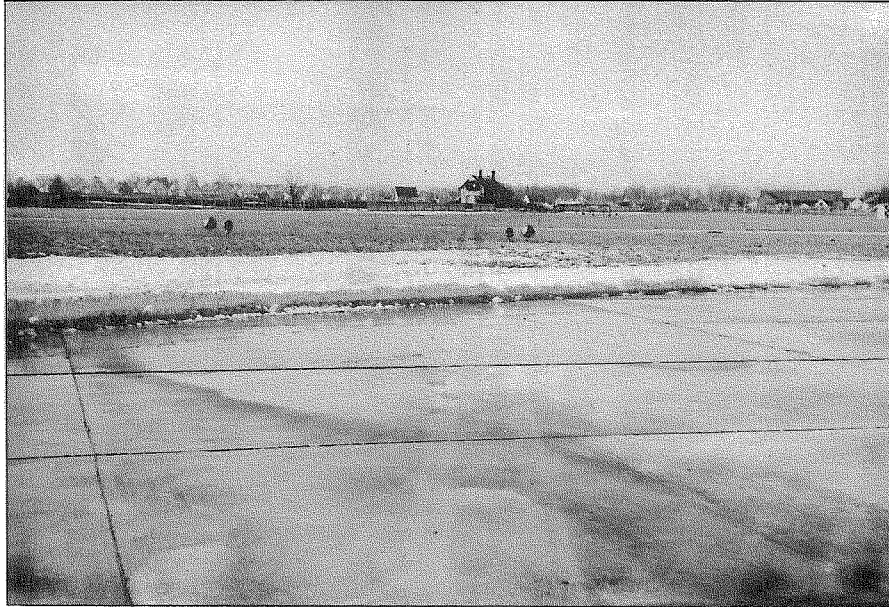
Fig. 9 Skid-marks left by right-hand undercarriage wheels at end of concrete runway.
