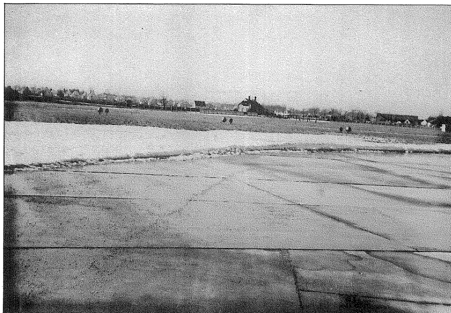
Fig. 10 Skid-marks left by left-hand undercarriage wheels at end of concrete runway.
