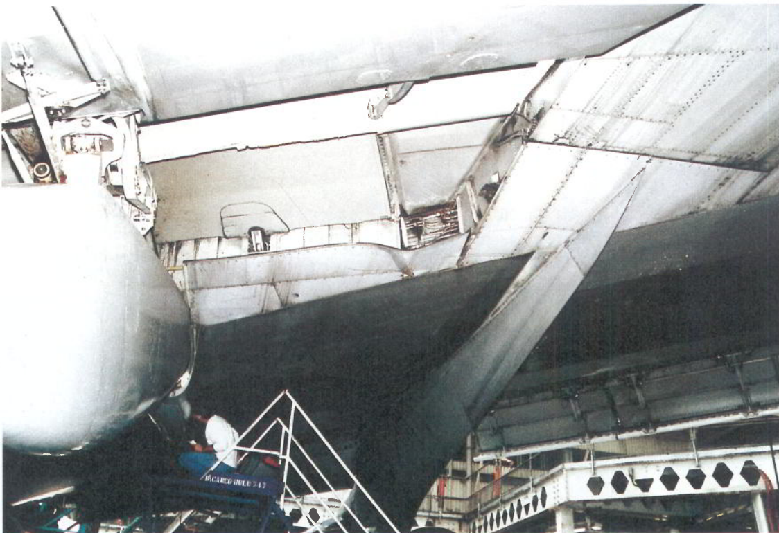
10. View of distorted wing panels outboard of no. 6 flap fairing
