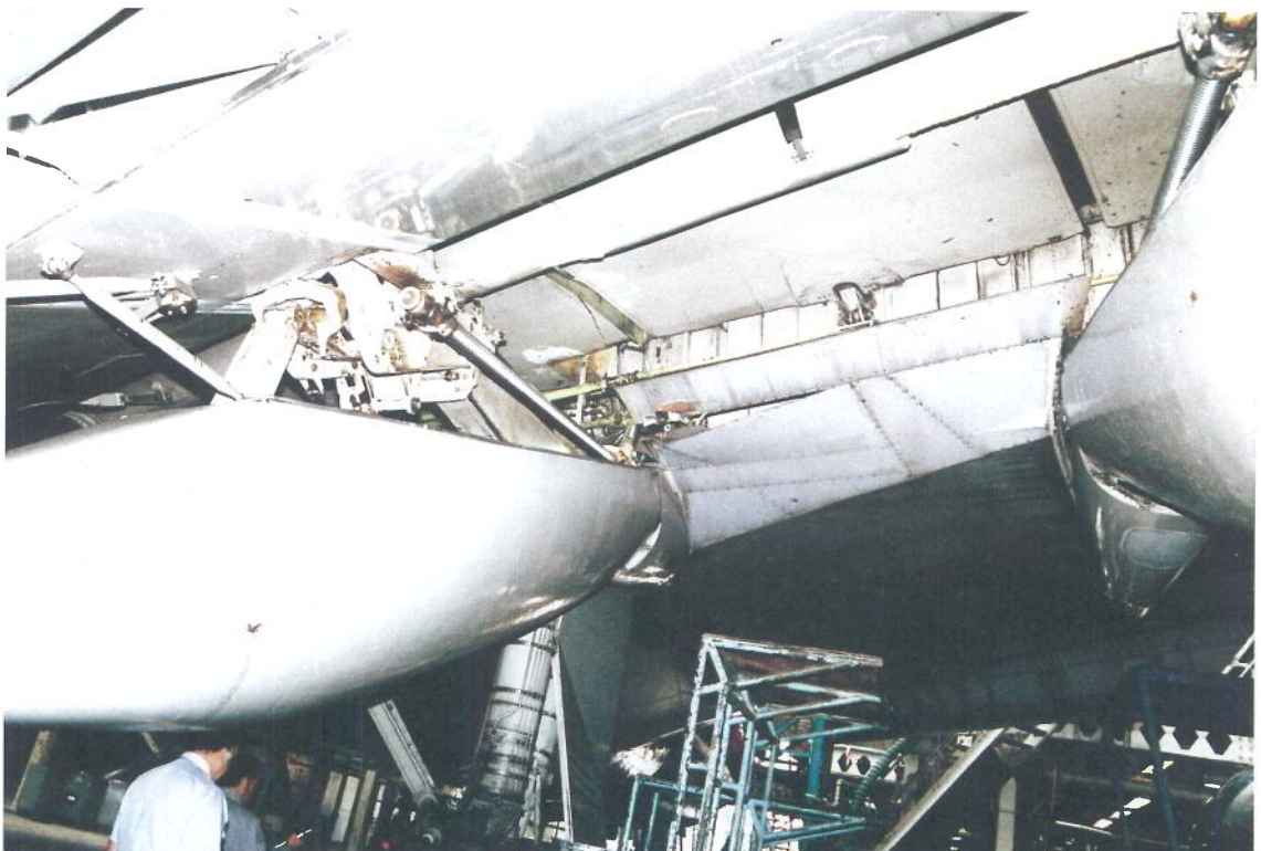
8. Showing damage to lower wing structure below spoiler support beam, adjacent no. 5 flap track
