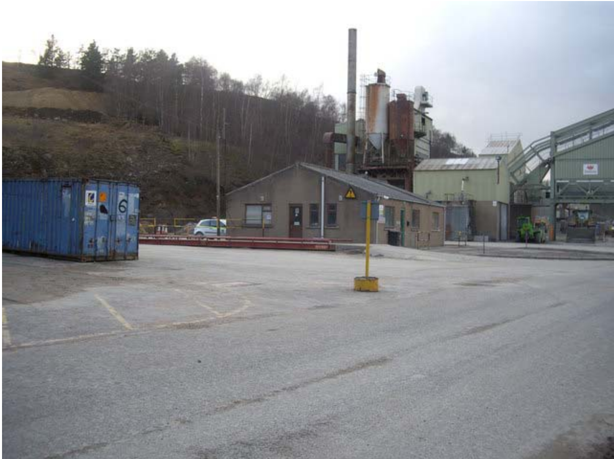
Aberdeenshire Council's Craiglash Asphalt Plant
