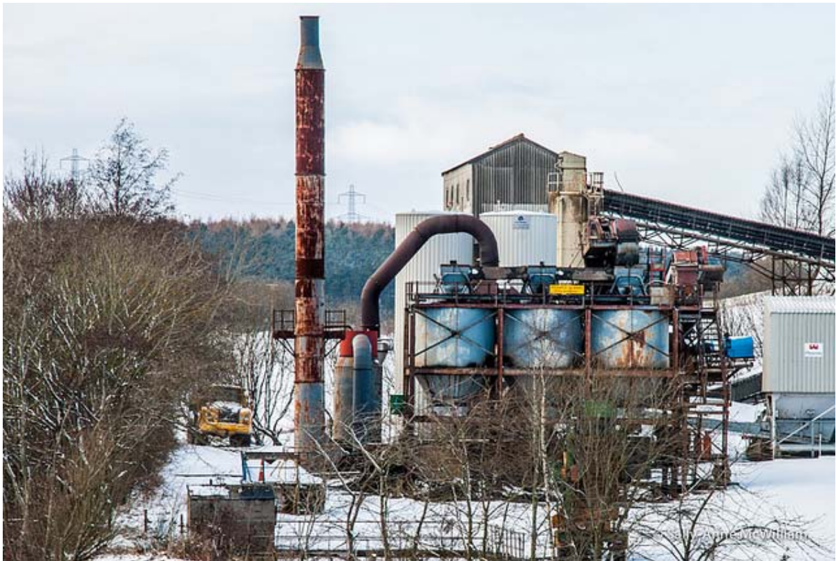
Aberdeenshire Council's Pitcaple Asphalt Plant
